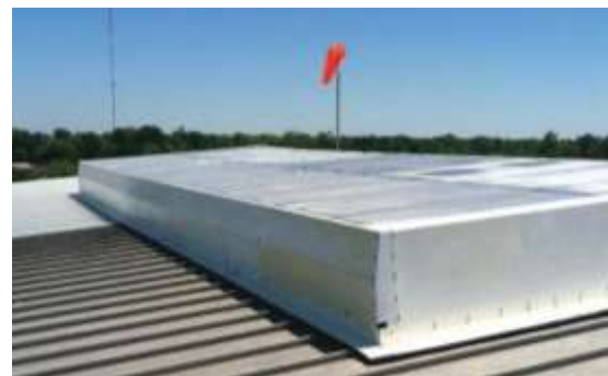
Labyrinth installed onto purlins, no roof curb.
