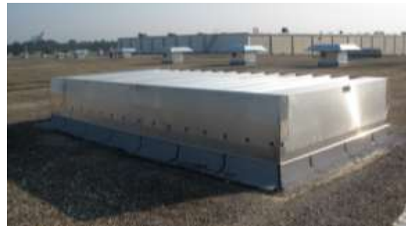
Labyrinth installed flat onto roof curb on a slanted roof.
