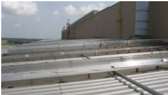
Labyrinth installed at an angle on a slanted roof.
