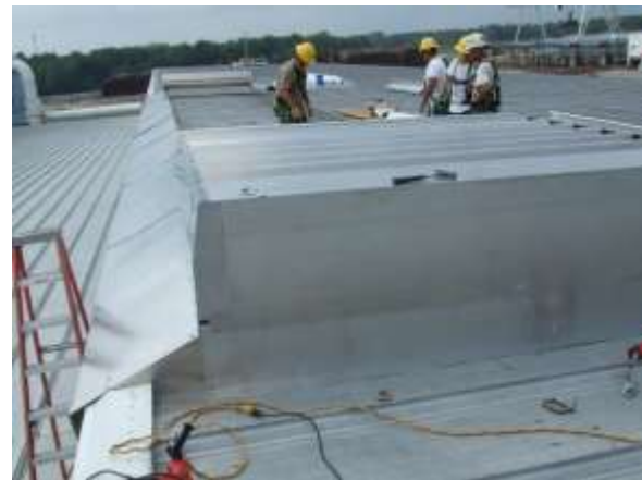
Labyrinth assembled directly on the roof of the facility
