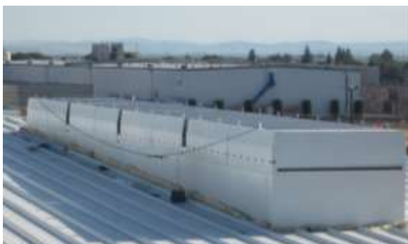
Labyrinth installed at an angle on a slanted roof.
