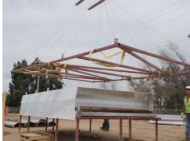
Ground assembly followed by lifting and roof installation
