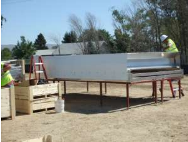
Ground assembly followed by lifting and roof installation
