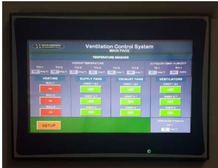
CoolStream Control Panel
