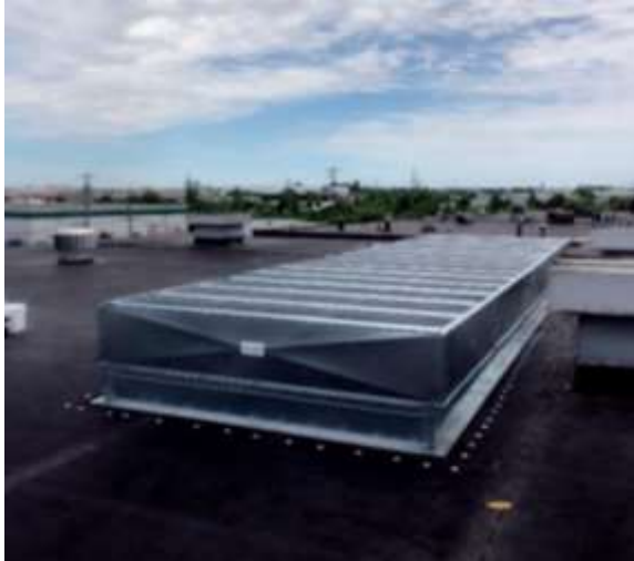
Flat Roof Mounted Thermoflow
