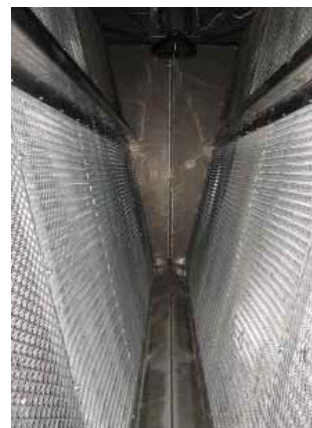
Draw through coil configuration.
