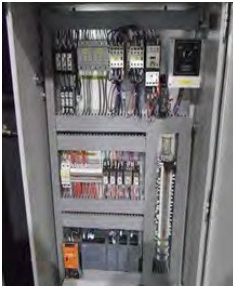
SEIMENS PLC WITH HMI
