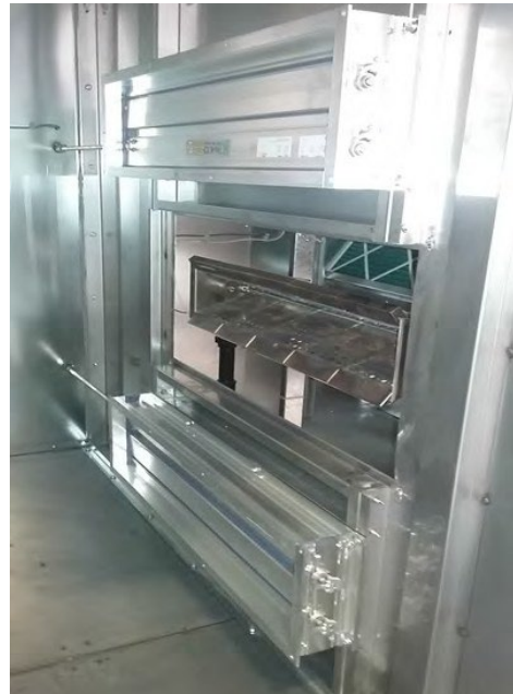
Bypass Damper with Burner
